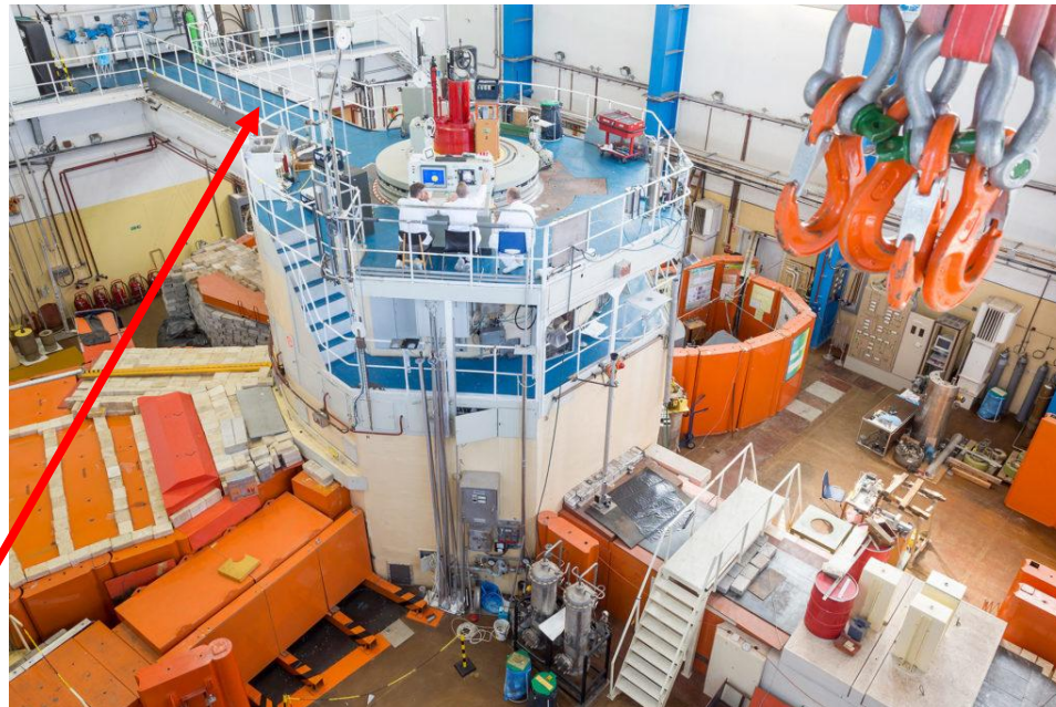
View from the corner of the room
